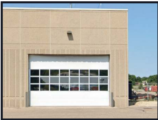
Fire Station 2 (Current) 22350 S Diamond Lake Rd. Rogers, MN 55374
