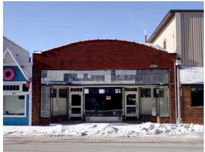
The City's former post office. Adaptive reuse can help grow its role as an asset to the City's built environment.
