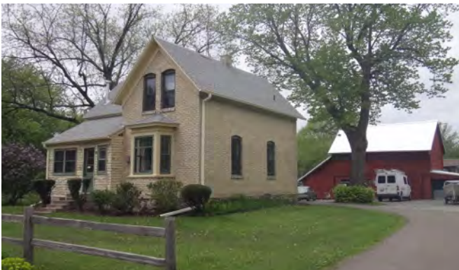
Brick home along Main Street in the "Outer Residential" sub-district.
