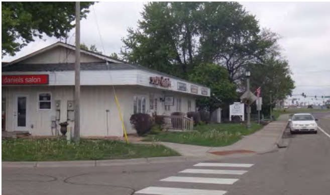
Commercial building at the “Edge of Main Street” district.
