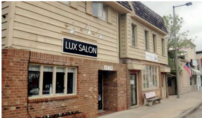
Heritage Main Street building covered in wood siding, with non-original mansard roof and brick veneer.
