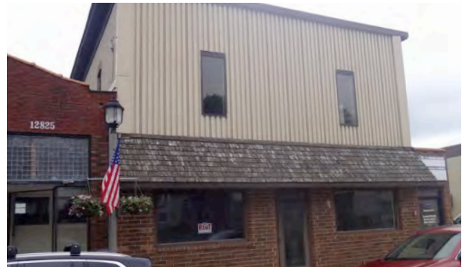
Two-story brick structure covered with metal sheeting in the "Heritage Main Street" sub-district.
