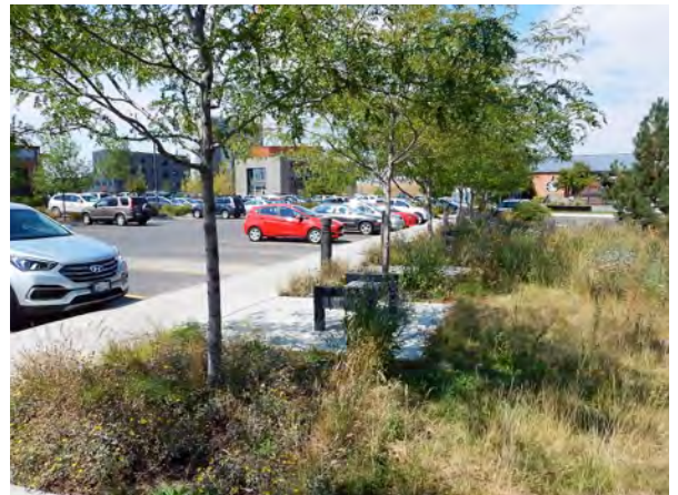
Stormwater feature to filter and detain runoff from parking area.
