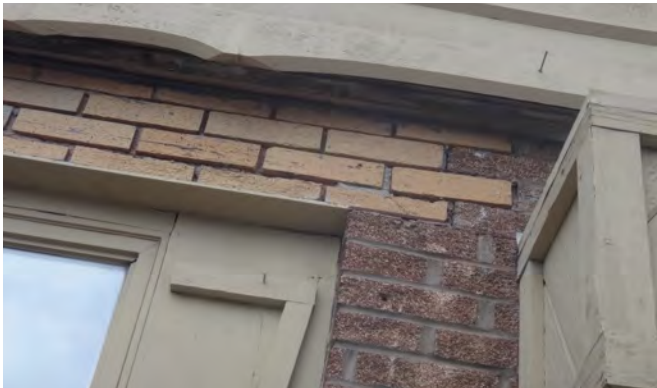
Modified / repaired lintel on a historic building along Main Street .
