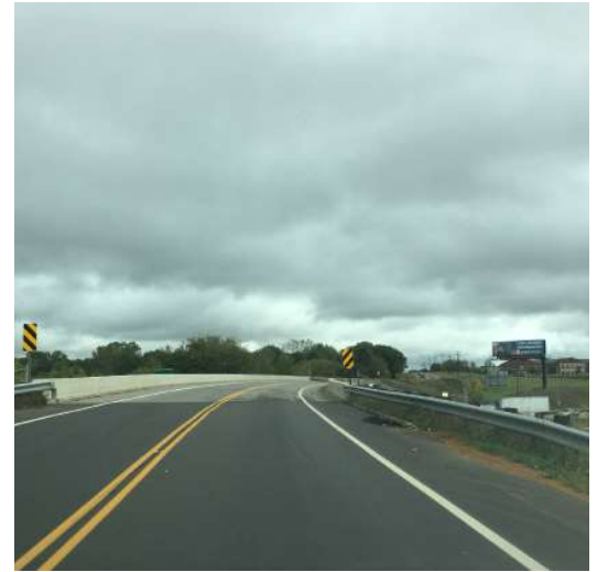
The existing bridge on 141st Avenue features a paved shoulder.
